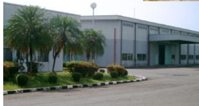
PT.Kawai Indonesia Plant 3
